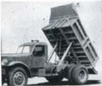
5. Dual Telescopic Hoist and Rock Body, Down Folding Gate.
